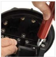
7.7 If required, using a locally-approved #6 bonding strap (not provided), connect the shield bond connector terminal to one of two bonding terminals located at the base of closure.
