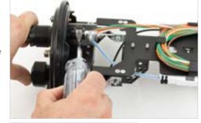
STEP 11: Closing Splice Closure 11.1 Reinstall the main closure gasket and apply a generous, even coat of high vacuum grease to ensure a water tight seal.
