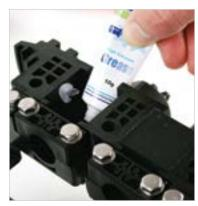
5.6 Install loop-thru or feeder cable and apply a generous amount of silicone sealant around the feeder grommet slit and cable sheath. Repeat for opposite cable port.
