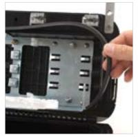
6.3 Remove the end grommet from the closure by pulling upwards, firmly. Cut the appropriate sized concentric cone of the grommet with shears.
