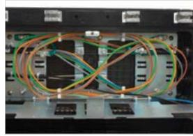
STEP 12: Installing Splice Trays
