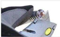
5. Install O-ring onto cable at third corrugation from jacket.
