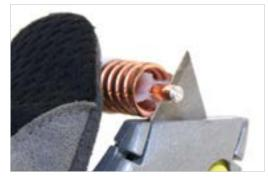
3. Install threaded gasket close to cable jacket.
