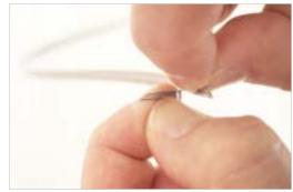
Carefully inspect the ribbon to determine if the split is in the center (between the blue and aqua fibers). If so continue to split the ribbon to the desired length. If not, repeat steps 1 through 4
