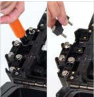
6.5 Remove the cable end grommet from the closure by firmly pulling upwards. Cut the appropriate sized concentric cone of the grommet with shears. Refer to Table 1 for diameters.
